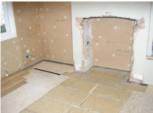
Internal: Pavatex ‘Pavadentro’ – 60mm, woodfibre boards, made from 95% waste soft wood. This was fitted to the internal walls front and back downstairs, with an overlap on side walls. When this insulation is added to 215mm brick, it gives a U value of 0.54 W/m<sup>2</sup>K.
