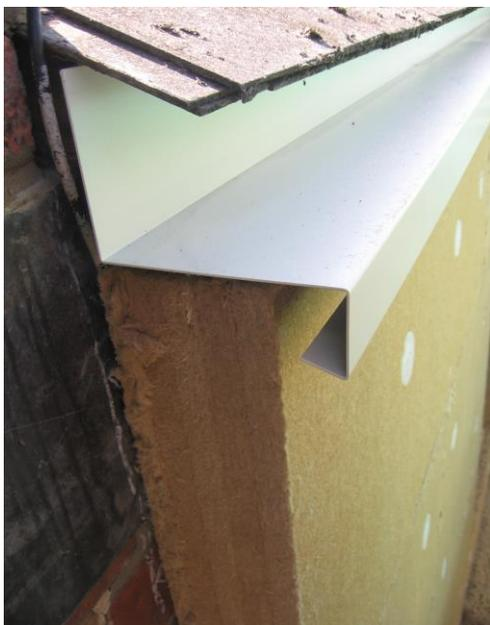
↑ Detail of soffit on top of insulation board before base coat and top coat applied. Gutters sit either on top or underneath soffit.
