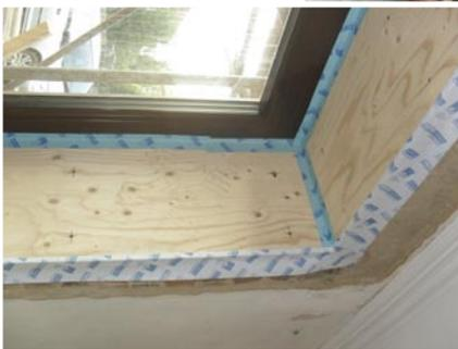
In this main photo we can see many of the details discussed in the design stage. The parge coat that was applied over the masonry; the external insulation and the detailing of the window boxes. The internal view of the window box can be seen in the inset photo above.
